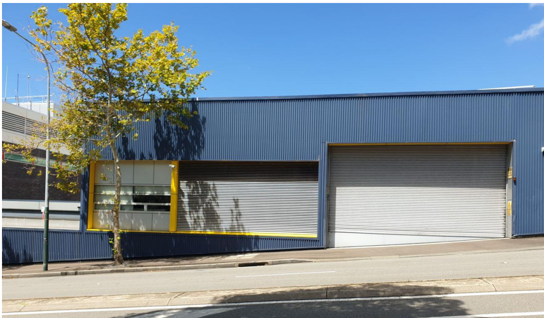
Figure 5: The Cross City Tunnel workshop site opposite at 80-94 Palmer St, Woolloomooloo, viewed from the western side of Palmer St, facing east
