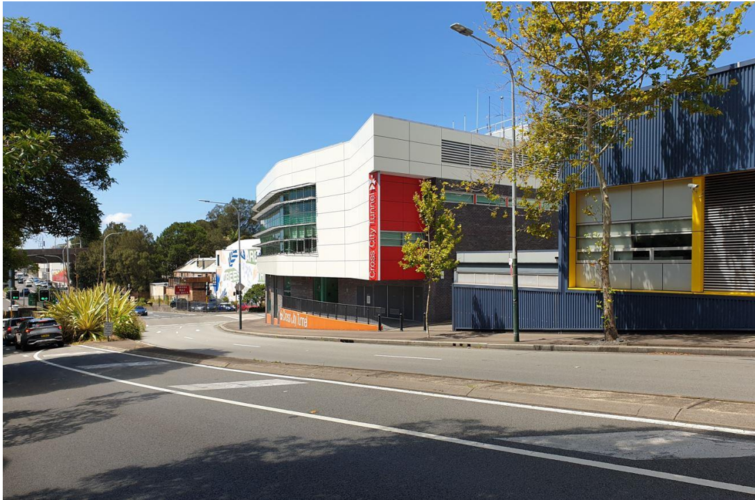
Figure 6: Cross City Tunnel administration building at 131 Cathedral St, Woolloomooloo, viewed from the western side of Palmer St, facing north-east
