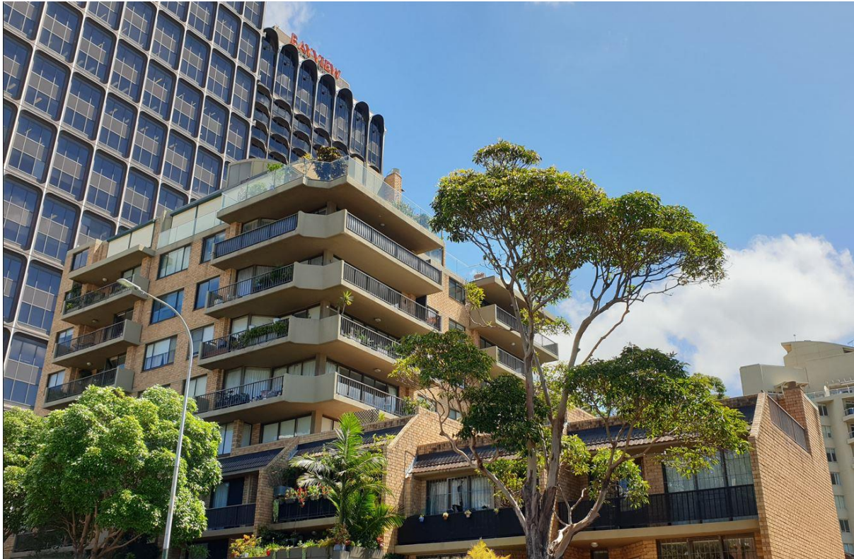
Figure 65: Photograph of the eastern (front) and northern (side) elevations of the apartment building at 113-125 Palmer Street, Woolloomooloo, viewed from the eastern side of Palmer St, facing south-west
