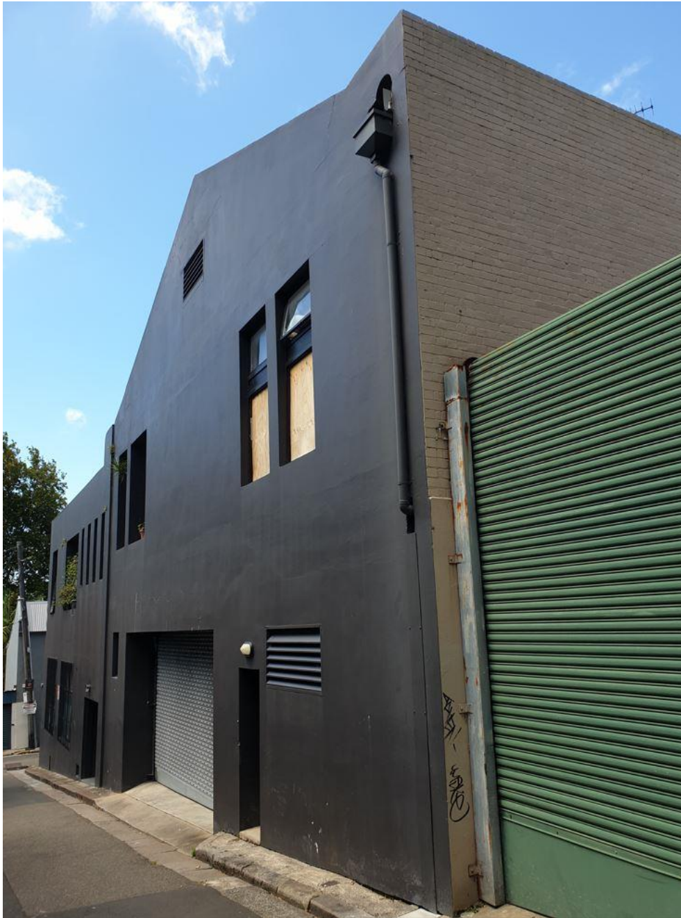
Figure 9: The rear of the adjoining site at 93-99 Palmer St, Woolloomooloo, viewed from the western side of Faucett Ln, facing north-east
